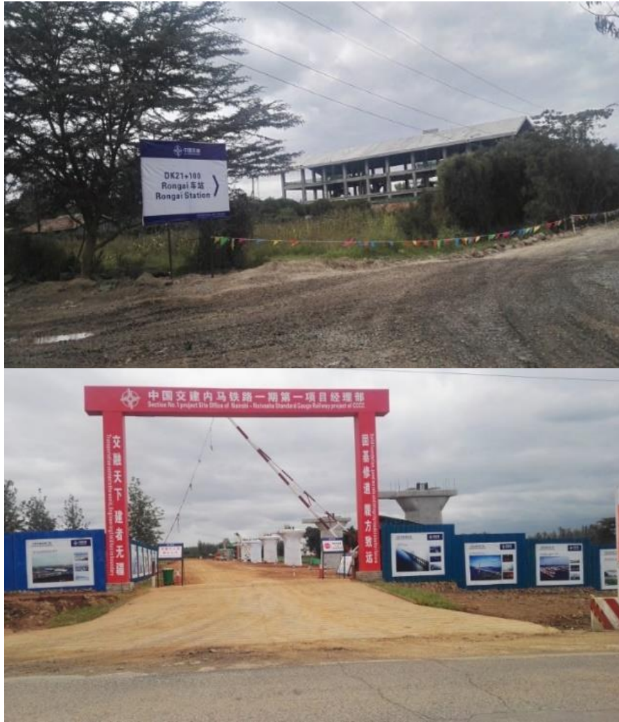
Image 3-4: Construction of the Kandisi and Ongata Rongai SGR stations (2018)
