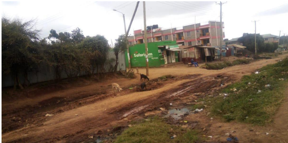
Image 3-2: Poor Road Condition at Gataka road
